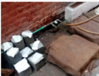
Curing of Concrete Test Samples
