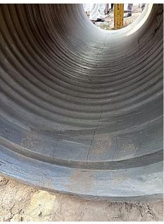
Figure 2: Cracking patterns.
