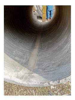
Figure 2: Cracking patterns.
