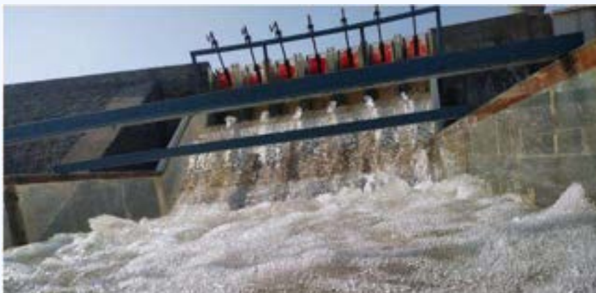
Air Bubble at Flow Surface of Upper Stilling Basin
