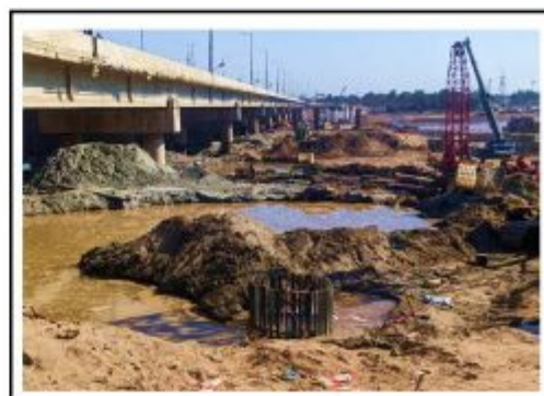
Field Image of Piles
